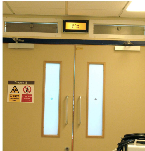
Figure 3: Illuminated Signs Displayed outside the Entrance to Theatre when X-Ray is in Use
